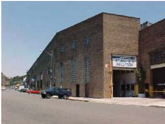
Photo: Industrial building facing White Bay
